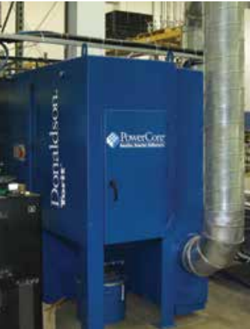
TG on Plasma Cutting 2,300 cfm (3,90 m³/h)
