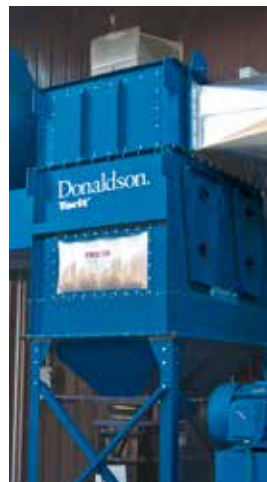
VH on Blasting 14,000 cfm (23,781 m 3 /h)
