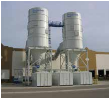
LP on Wood Dust 160,000 cfm (271,784 m 3 /h)
