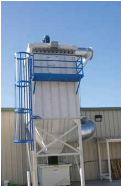
FS on Woodworking 20,000 cfm (33,973 m 3 /h)
