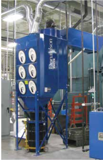
DFO on Rubber Grinding 2,500 cfm (4,247 m 3 /h)
