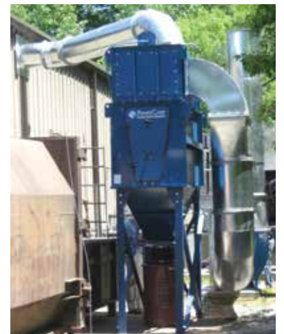
VH on Grinding 9,000 cfm (15,288 m 3 /h)
