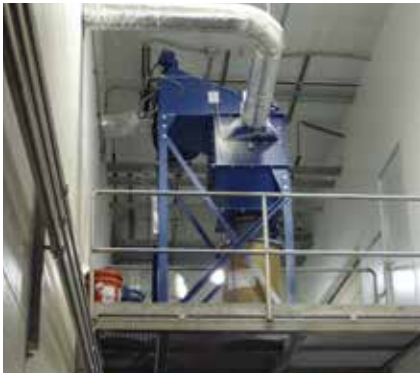
CPC on Milk Powder 1,200 cfm (2,038 m 3 /h)
