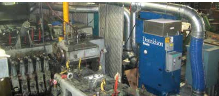
WSO on Cold Forming 1,200 cfm (2,038 m³/h)
