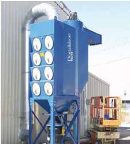
DFO on Plasma Cutting 5,000 cfm (8,493 m³/h)
