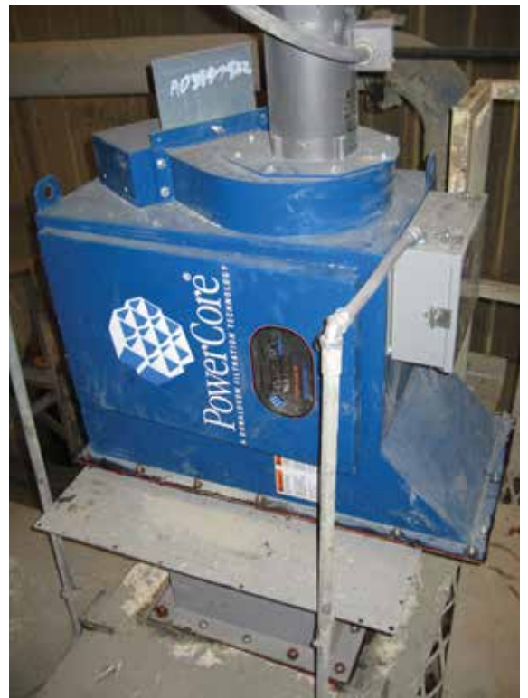
CPV - Feed Hopper 350 cfm (595 m 3 /h)
