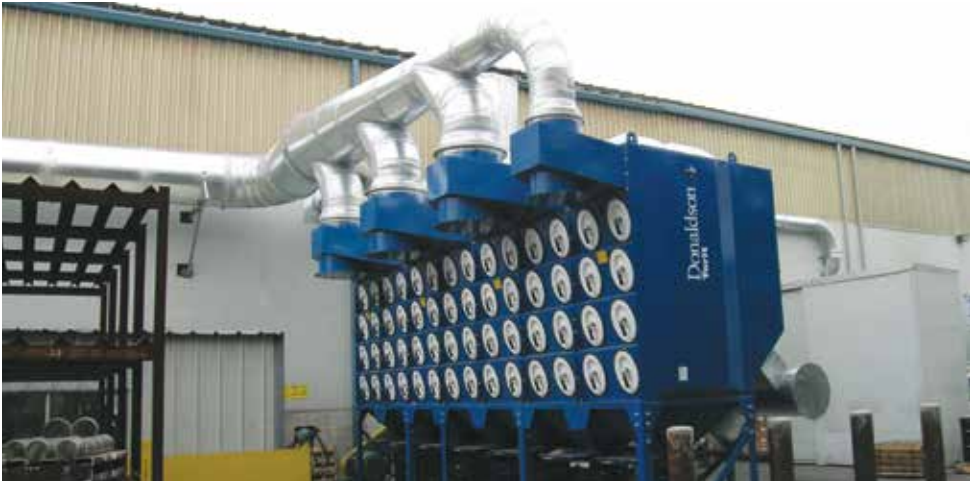
DFO on Grinding 74,000 cfm (125,700 m³/h)
