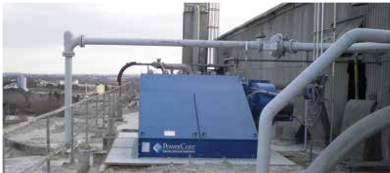
CPV - Multiple Cement Silos 4,800 cfm (8,154 m 3 /h)
