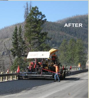
"Your Warm Mix Asphalt was consistently processed at 240-250° F and the hand work was just as easy as hot mix asphalt."
